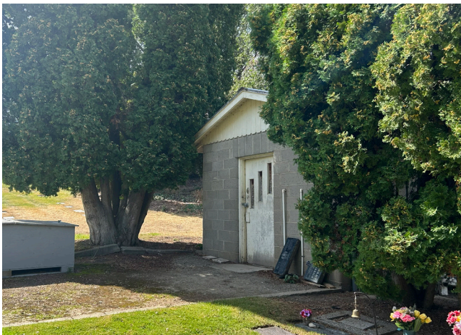
Figure 12: Maintenance and Storage Shed, Source: LEES+Associates.
