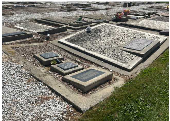
Figure 15: Cracked and Sinking Concrete Vaults in Older Sections of the Cemetery, Source: LEES+Associates.
