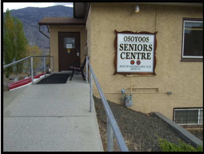
Photo 99: Osoyoos Seniors Centre – Accessible ramp and automatic door opener
