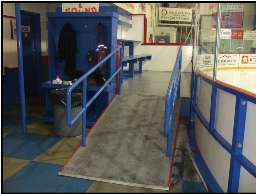
Photo 23: Sun Bowl Arena – Accessible viewing area
