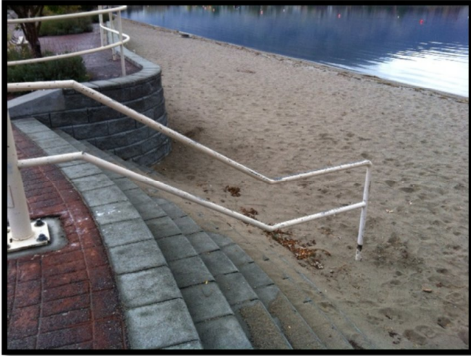
Photo 48: Cottonwood Park – Staircase
