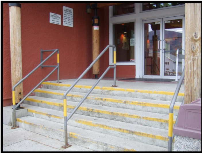
Photo 8: Sonora Centre – Staircase by north entrance
