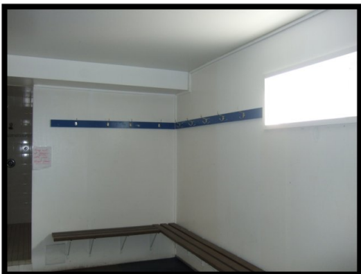
Photo 31: Sun Bowl Arena – Example of inaccessible coat hook rack
