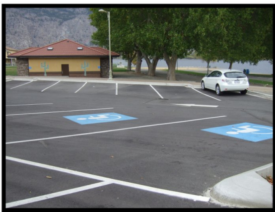
Photo 57: Gyro Park – Parking stalls on cross slope
