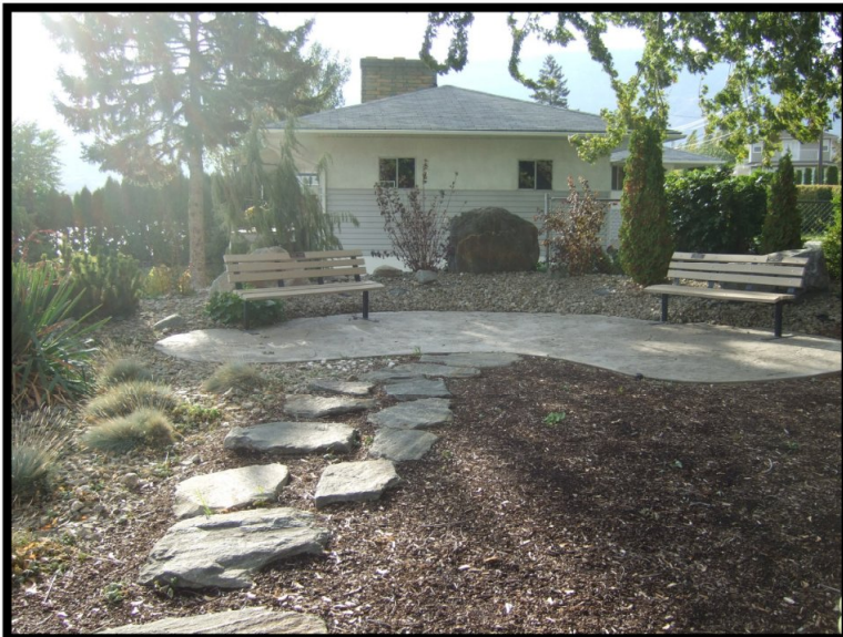
Photo 83: Veterans Park – Inaccessible pathway
