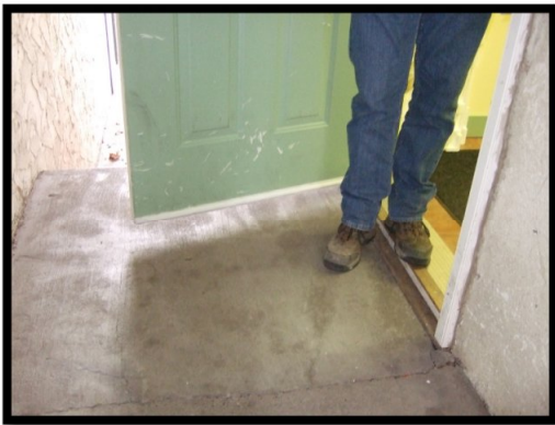
Photo 39: Planning and Development Services – Small level threshold area at top of ramp
