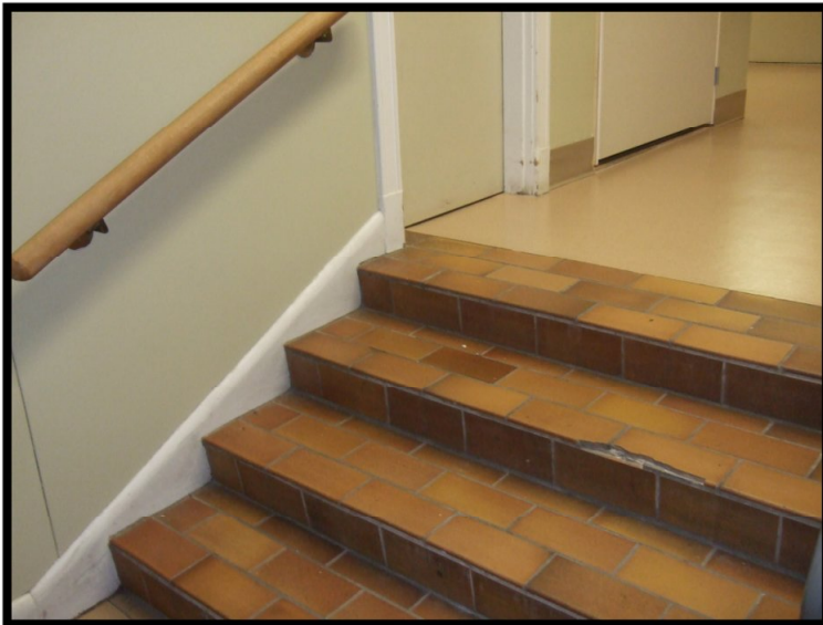
Photo 5: Sonora Centre – Stairway by east entrance
