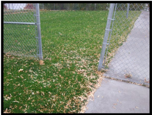
Photo 2: Sonora Centre – Inaccessible pathway from parking lot to basketball court
