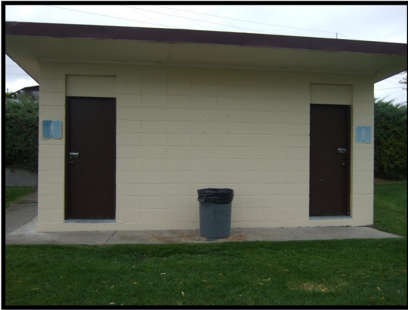
Photo 68: Legion Beach – Washrooms with front step
