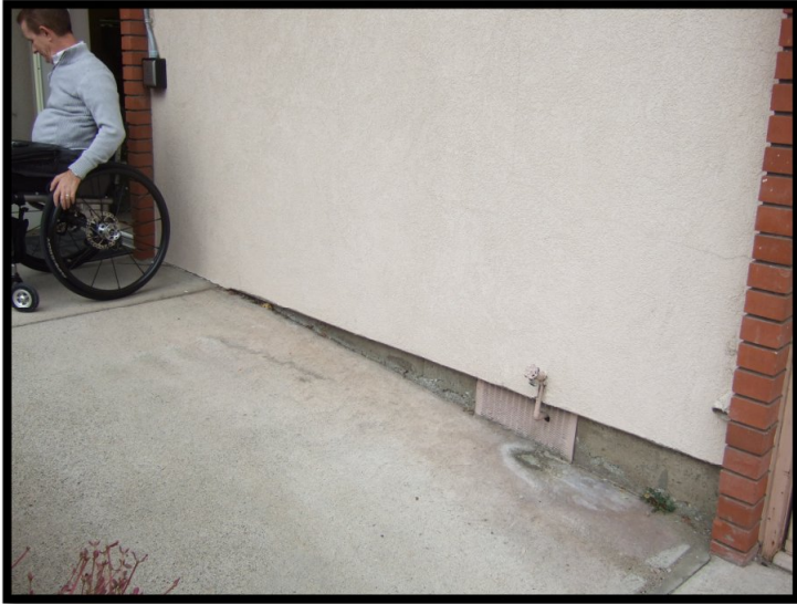
Photo 36: Town Hall – Upper portion of ramp leading to Council Chambers
