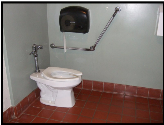
Photo 12: Sonora Centre – Inside of accessible washroom
