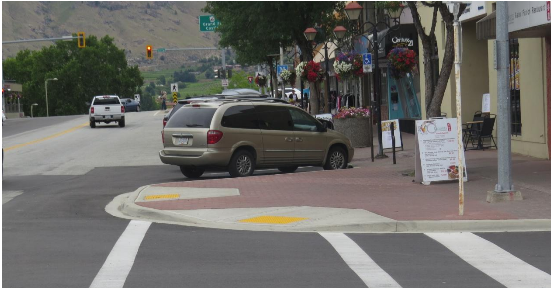
Existing Sidewalk Extension (bulge) on Main Street
